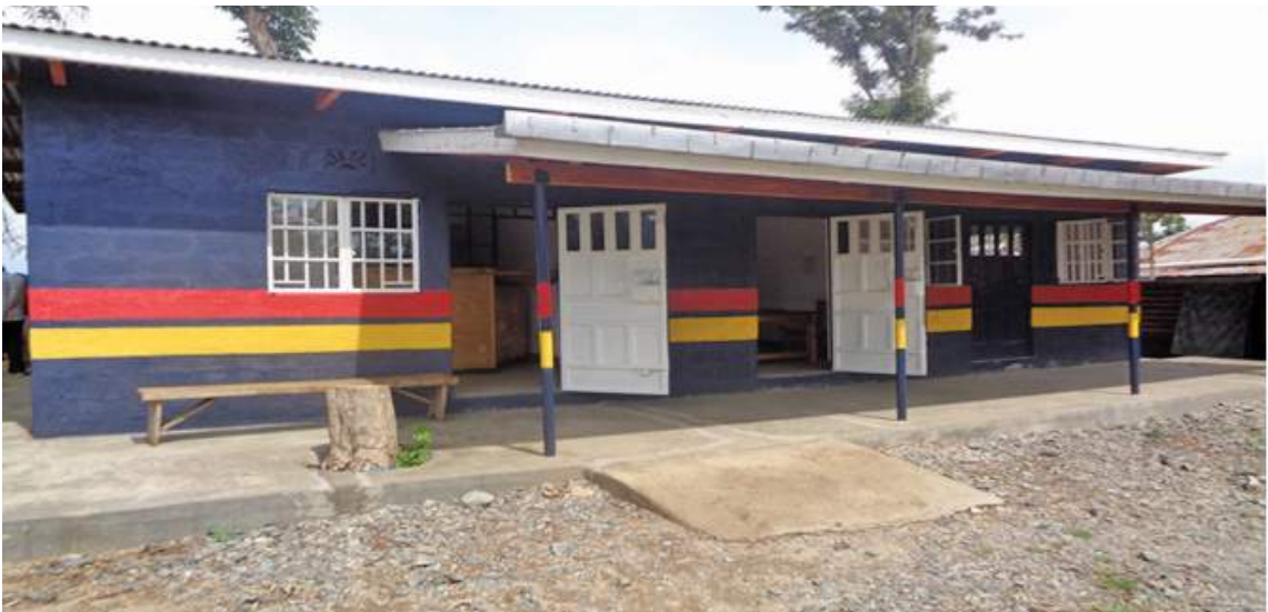
Figure 20; Chemase Patrol Base at follow-up inspection in February 2018.
