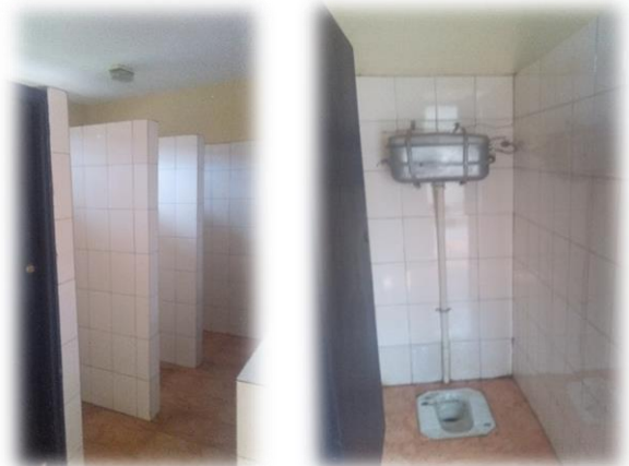
Clean Cell showers and toilet at Lumakanda Police Station
