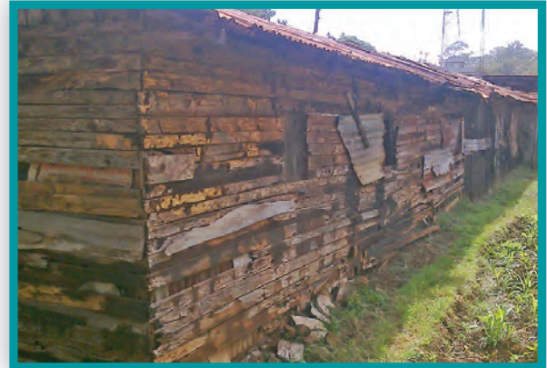
Police accommodation at Kerugoya Police station
