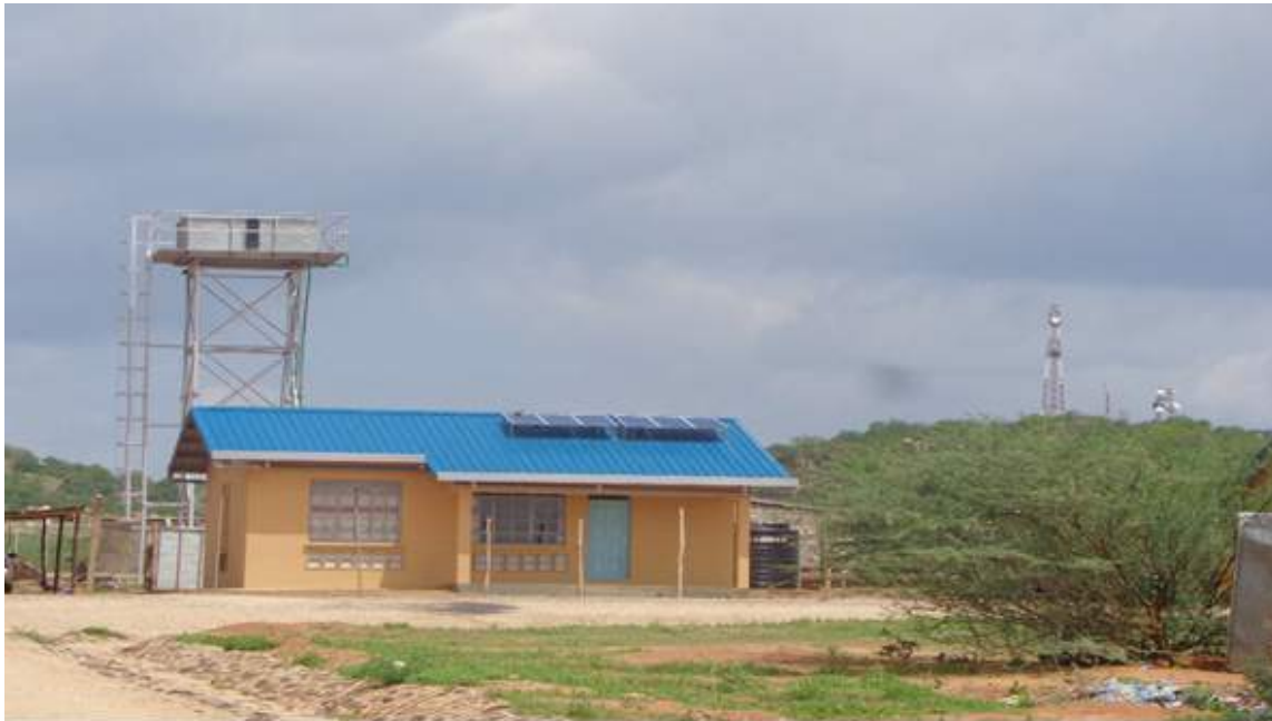
Nov 2017; newly constructed police houses at Turbi Police Station in Marsabit County.
