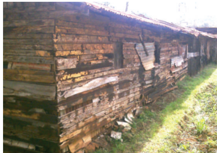
Police accommodation at Kerugoya Police station
