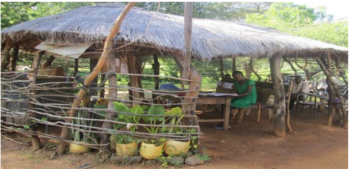
Figure 5: A grass thatched structure used as a Report Office at Gatunga Police Station, Tharaka Nithi County. Source: (IPOA, 2020)
