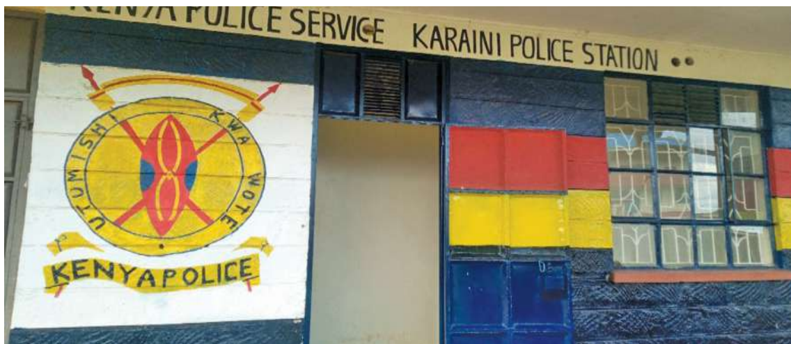
Photo 1: A renovated office block at Karaini Police Station
