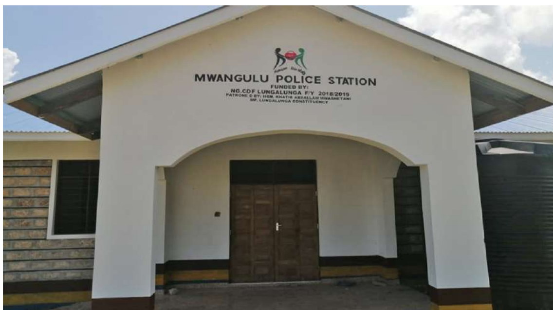
Photo 1: Offices under construction at Mwangulu Police Station, which are funded by NG-CDF Lungalunga
